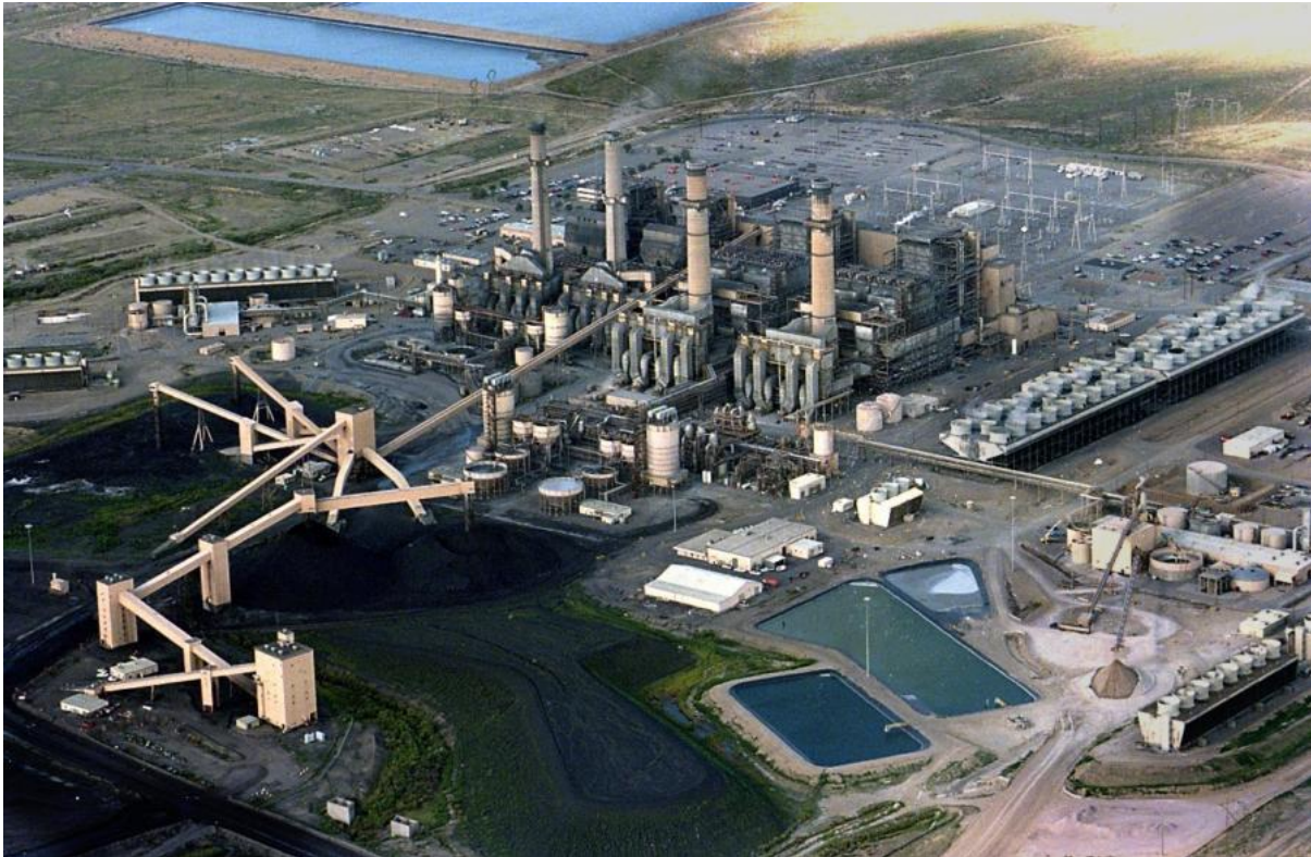
The San Juan Generating Station. (Richard Pipes/Albuquerque Journal)
