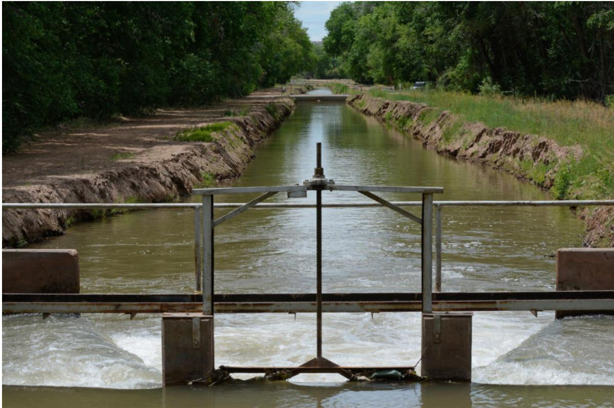
A diversion gate that feeds the acequias in the North Valley is pictured. The Middle Rio Grande Conservancy District operates and maintains many miles of laterals, ditches, canals and drains used to convey water to and from cropland. The district is holding a board election June 6. (Jim Thompson/Albuquerque Journal)
